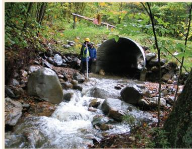
◀A recently installed arched culvert designed with the Stream Simulation Approach on the Green Mountain National Forest days after the Hurricane Irene catastrophe shows no stream blockage. USDA Forest Service photo.
